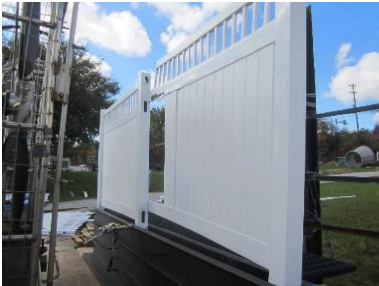
Photo No. 4 Fence Failure / Configuration 2 - Mason
