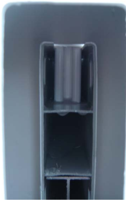
Photo No. 1 Horizontal View through Post Routing Showing Inserted End of Bottom Rail, Groove Side of First Picket and Aluminum Reinforcement
